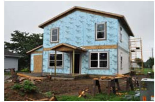
Habitat home in Iowa City under construction in 2009
